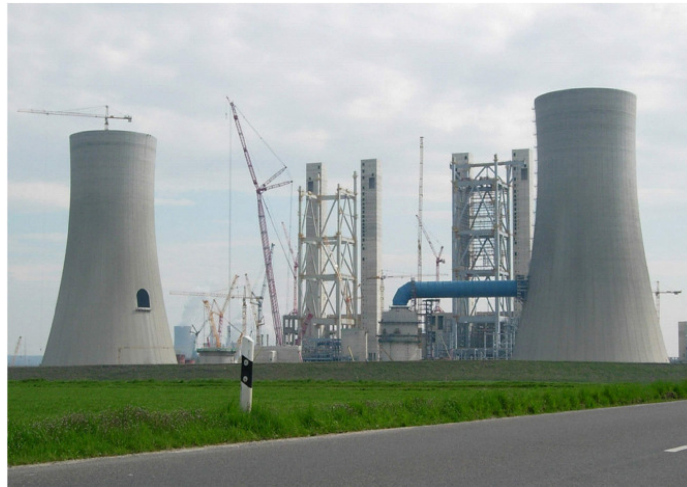
Figure 10: RWE double blocks at Neurath under construction in summer 2007
