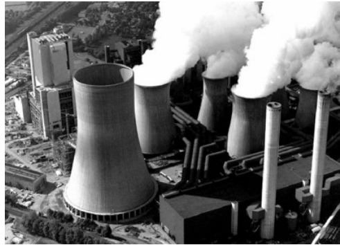
Figure 1: RWE Power Station Niederaussem under construction in 2001 (Photo RWE)
