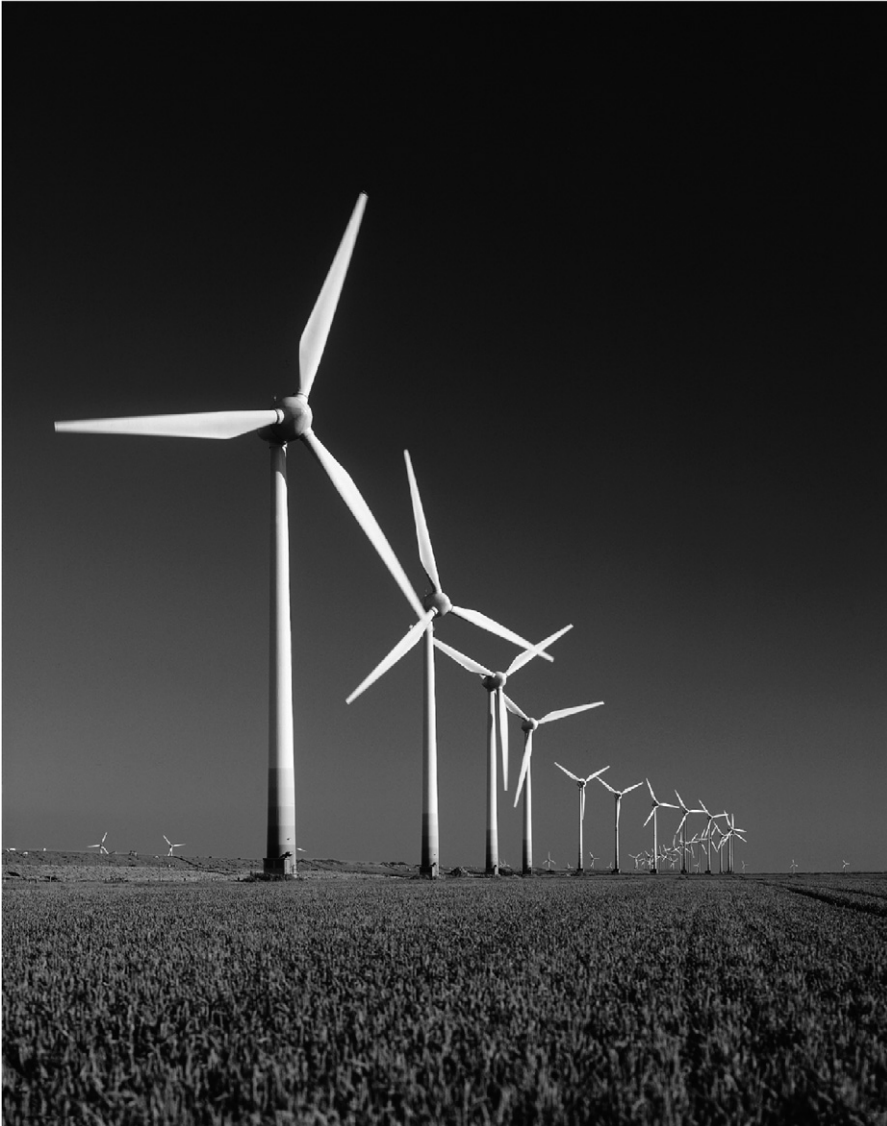
Fig. 3. Steel tube towers (Enercon).
