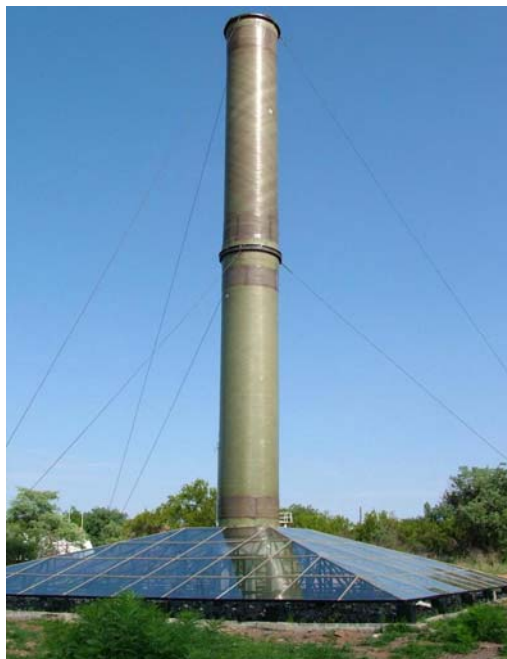
Figure 1. Solar Chimney Installed at BOTEC headquarters.
